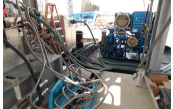
Process Equipment Set Up
