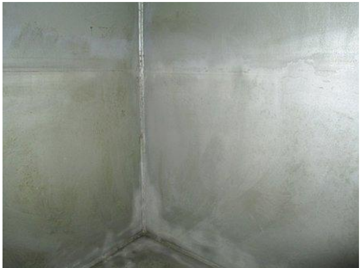
Reservoir walls after cleaning
