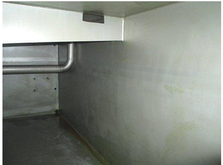
Reservoir Floor After Cleaning
