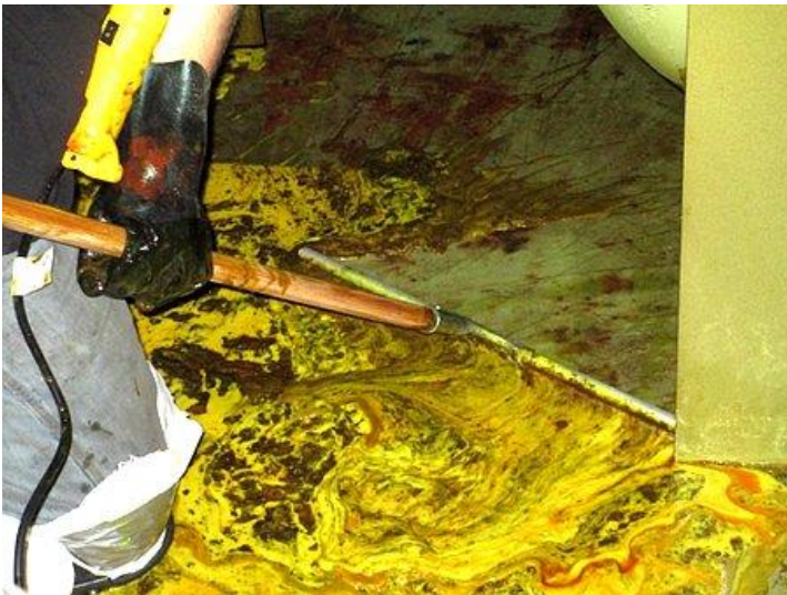
Reservoir sludge removal before cleaning
