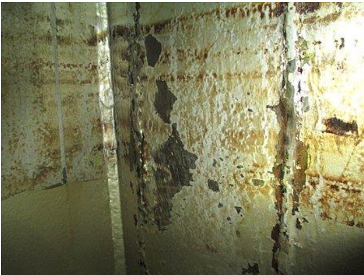
Reservoir walls before cleaning
